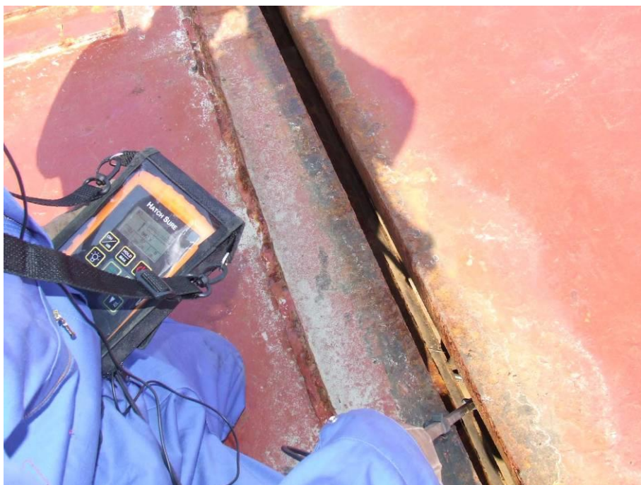
Fig 7.8. Scanning a Deep Hinged Joint.
