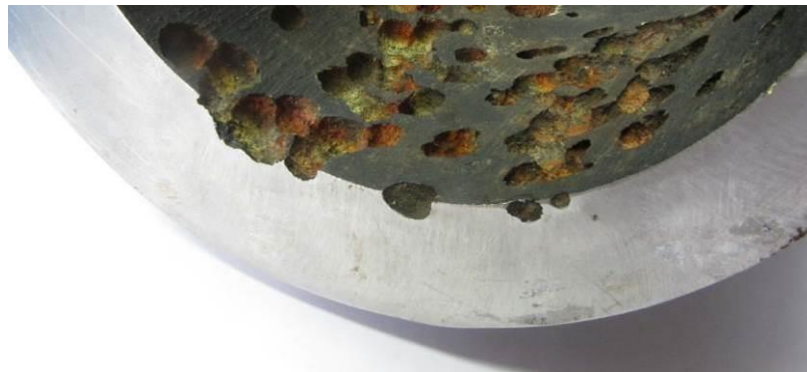
Large Corrosion Pits.
